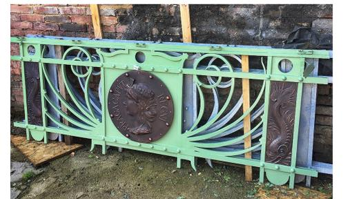
Application of corrosion protection to railing segment of the bridge of Svatoopluk Čech
