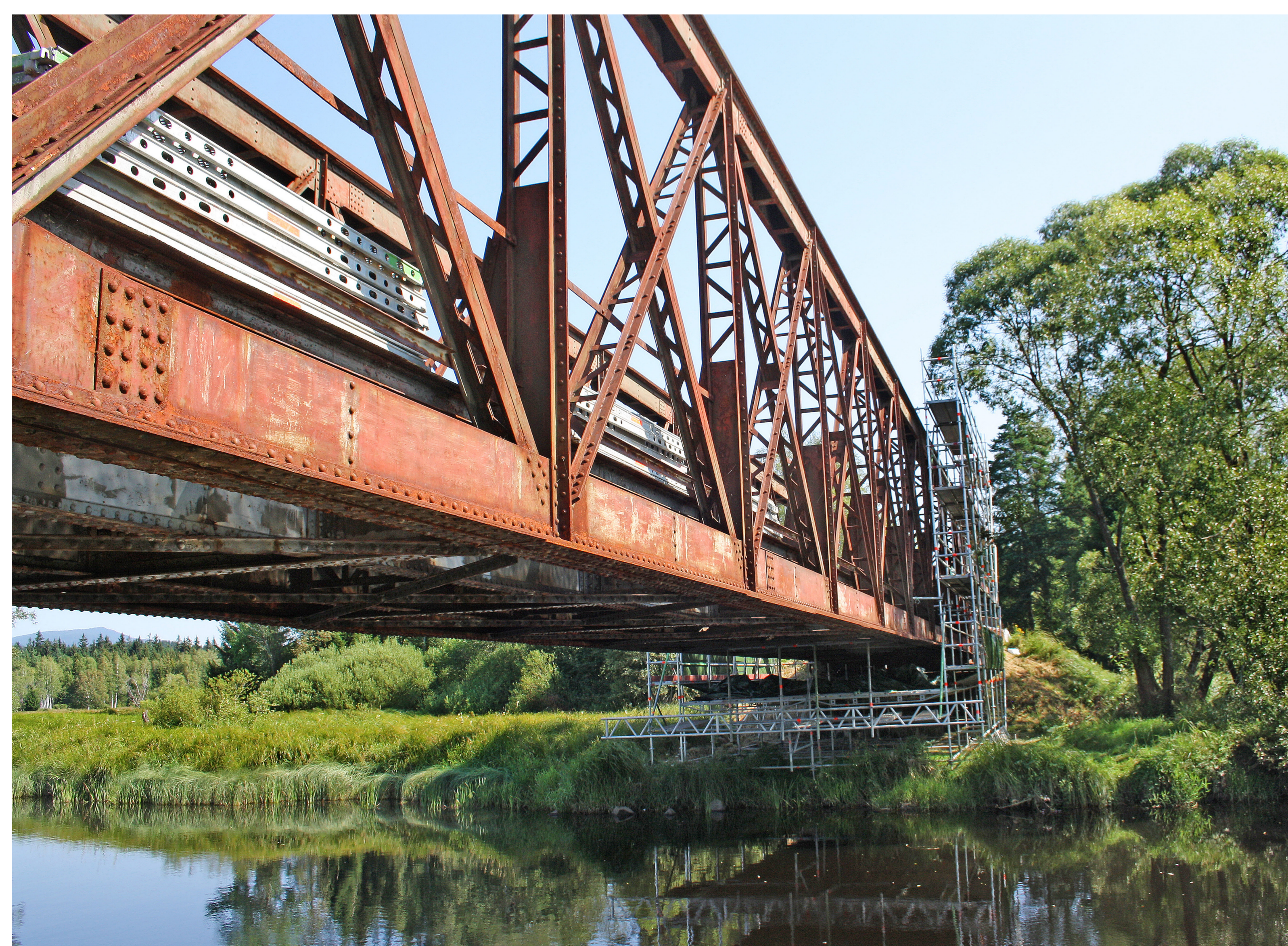
Protection of the Komenský Bridge in Jaroměř by hot-dip galvanizing, 2015
