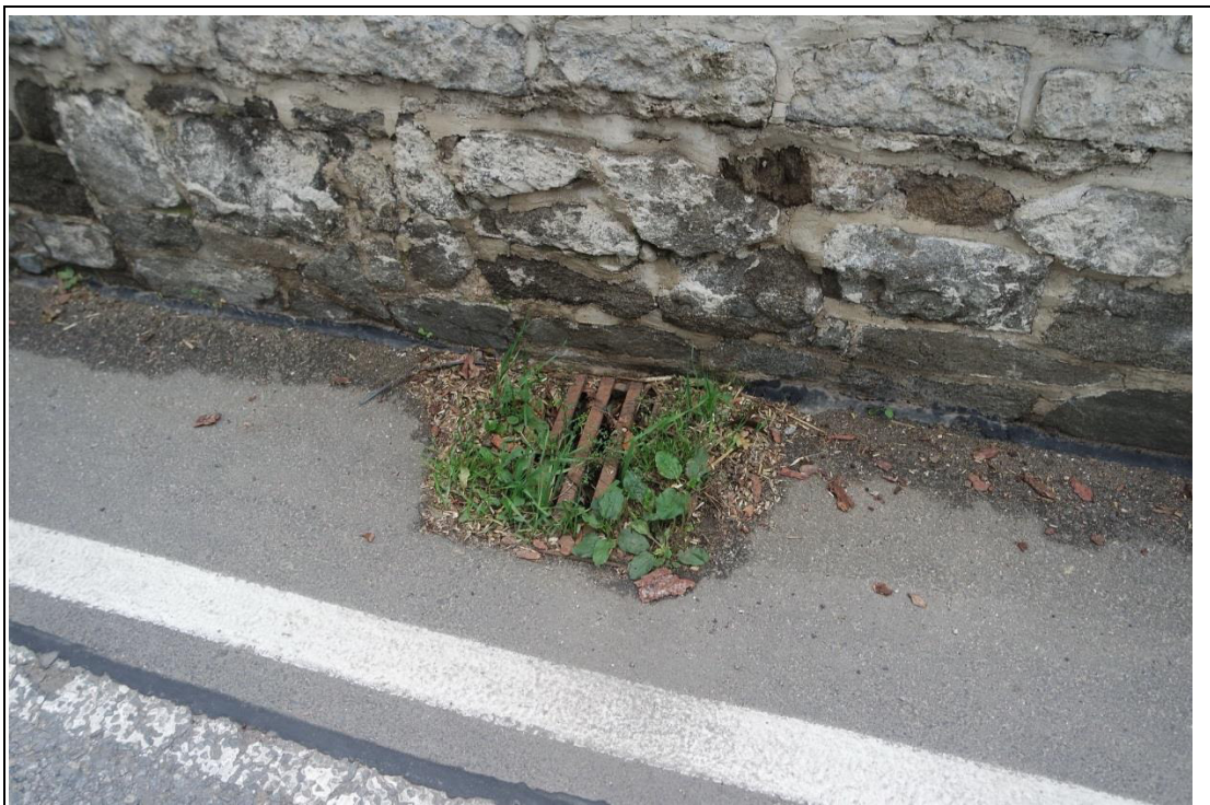
Fig. 30 Block drainage (upstream side)
