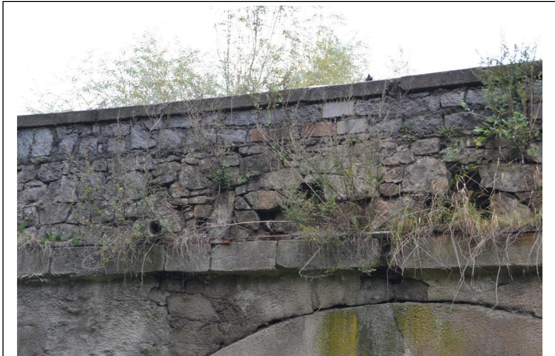
Fig. 27 Plant vegetation on the parapet (downstream side)
