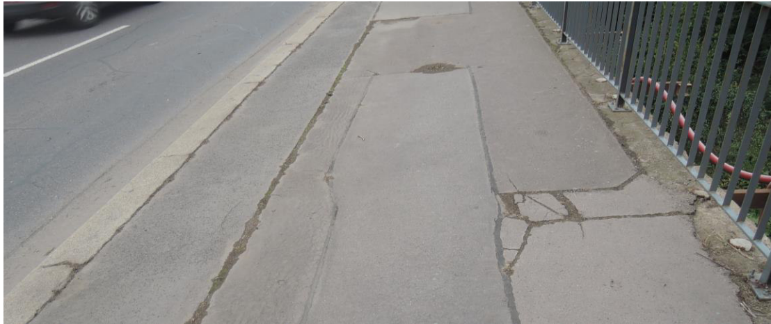
Figure 2.2-11 - Denivelation of the pedestrian walkaway
