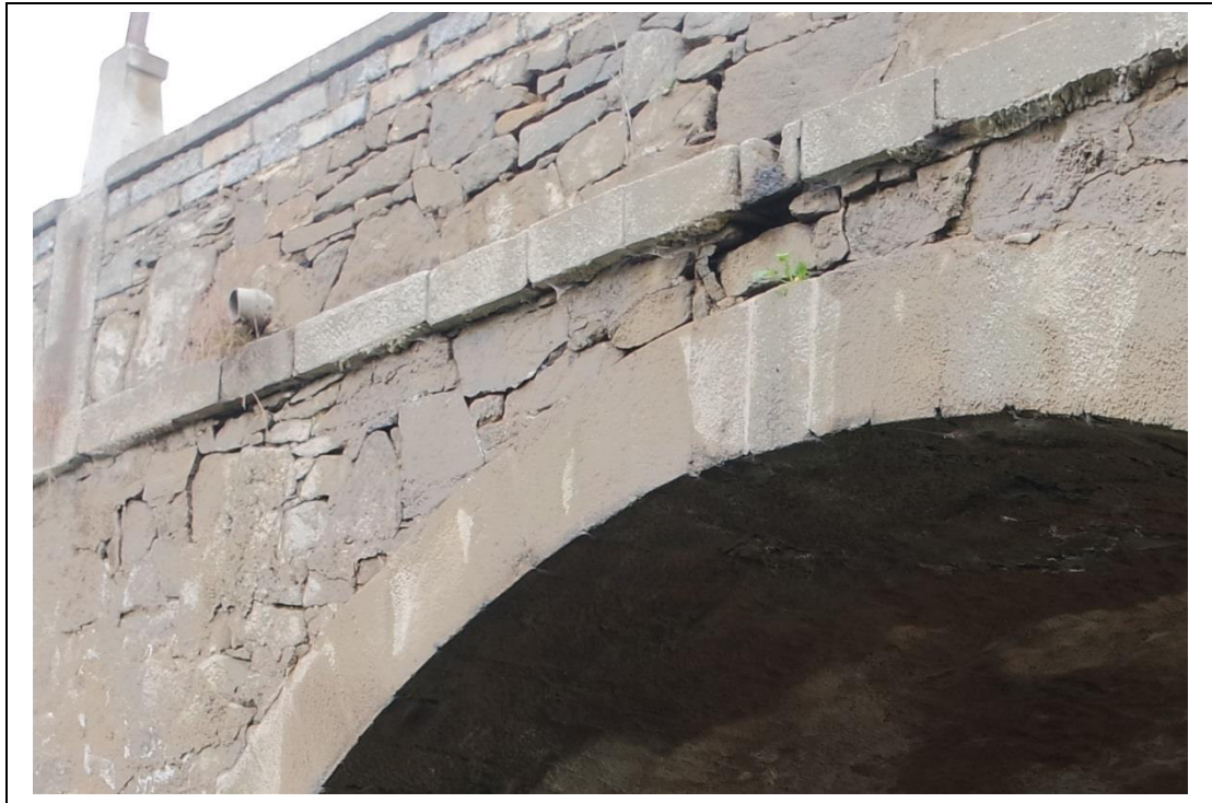
Fig. 19 Loss of mortar in spandrel wall (upstream side)
