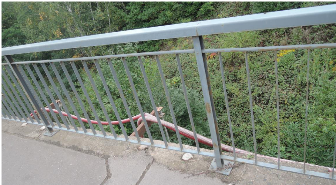
Figure 2.2-15 – New bridge railing
