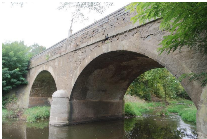
Fig. 2 Side view of the bridge (upstream side)
