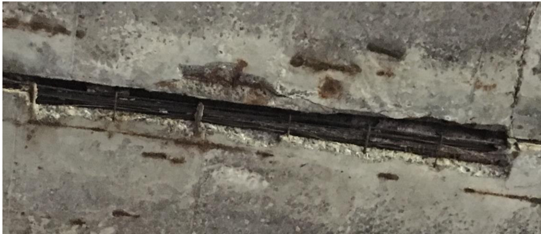
Figure 2.2-4 - Girder G11 with visible tendons
