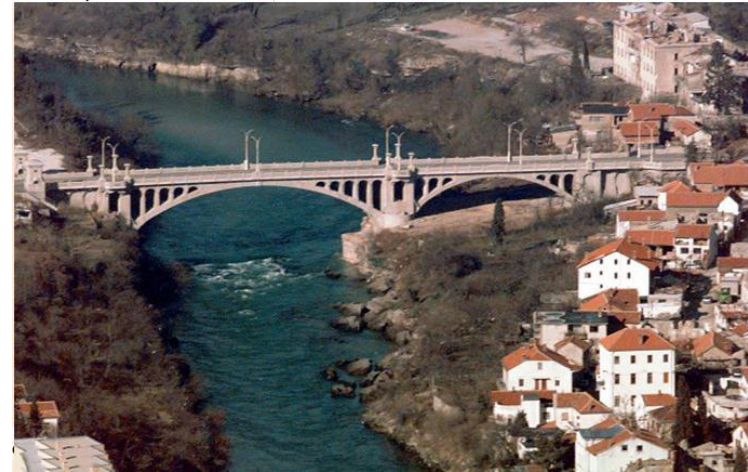
Arch Bridge Carinski most, Mostar Bridge Bosnia and Herzegovina
