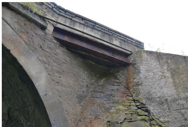
Fig. 6 Widening of the bridge
