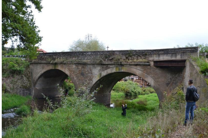
Fig. 1 Side view of the bridge (downstream side)
