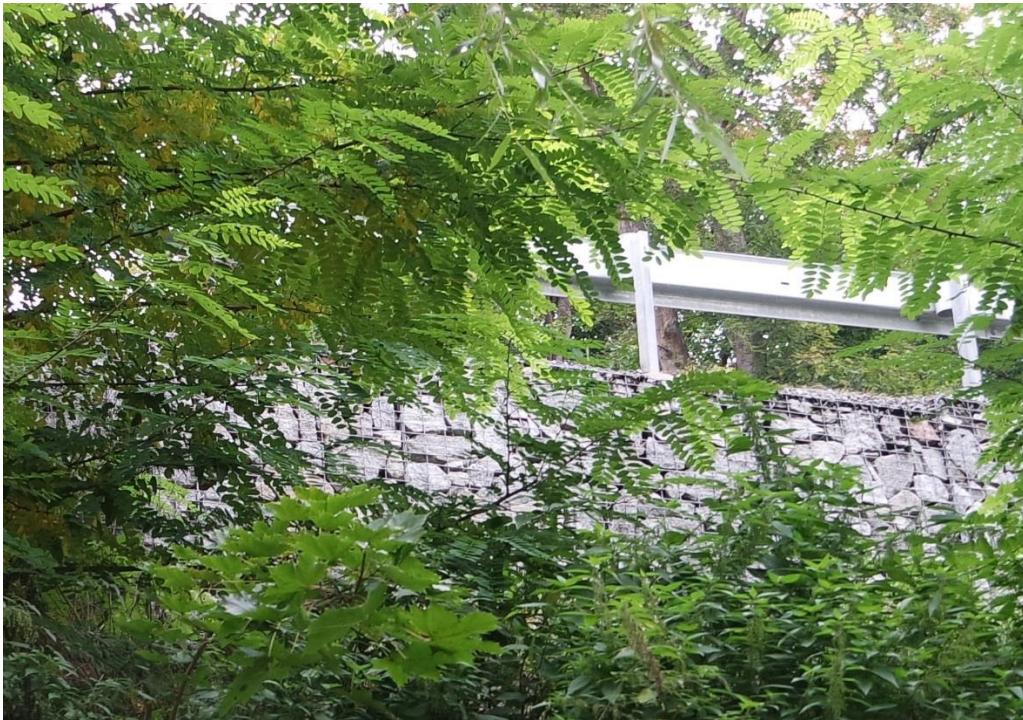
Fig. 8 Gabions on the embankment of the bridge
