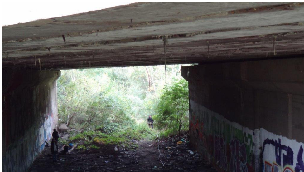
Figure 1.1-2 - General overview of the Kolbenova bridge substructure
