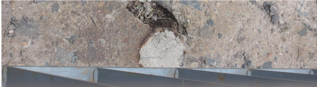
Figure 2.2-14 - Anchorage of removed railing
