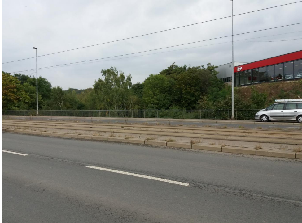
Figure 1.1-1 - General overview of the Kolbenova bridge superstructure
