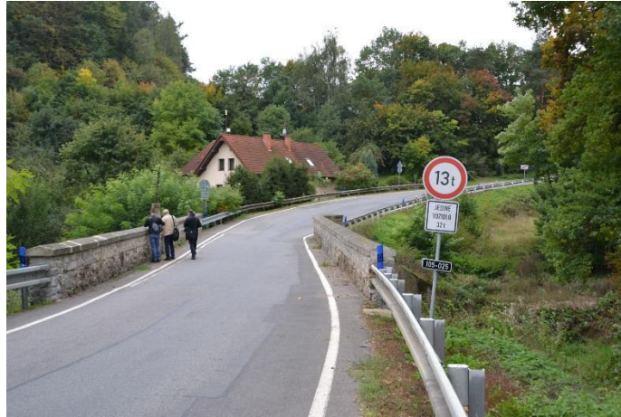
Fig. 4 A view along the road from the right side of the bridge
