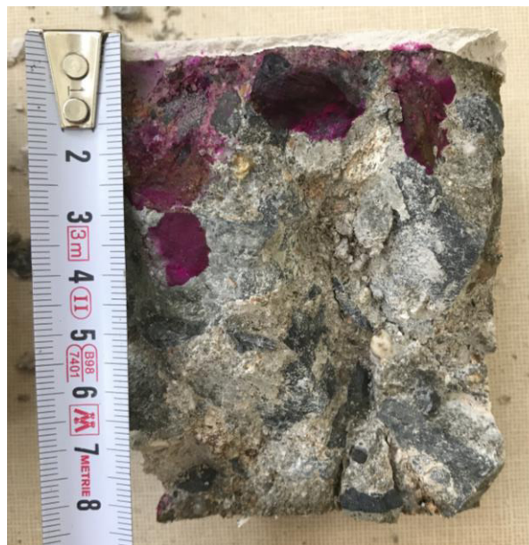
Figure 3.2-1 - Carbonation of the main girder core
