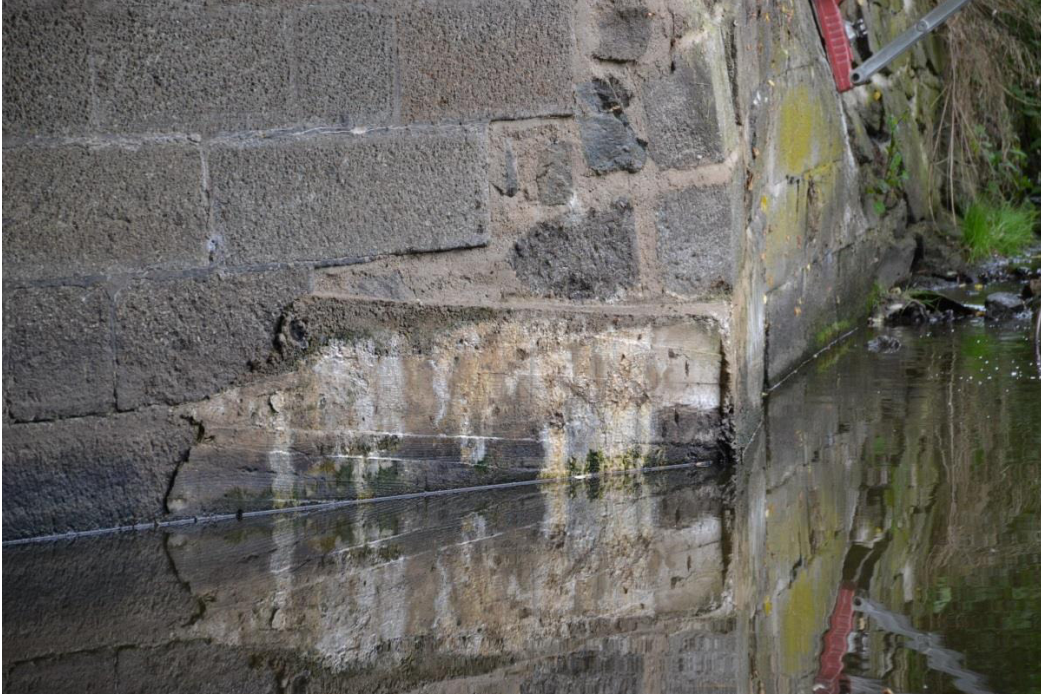
Fig. 7 Repaired part of abutment 3
