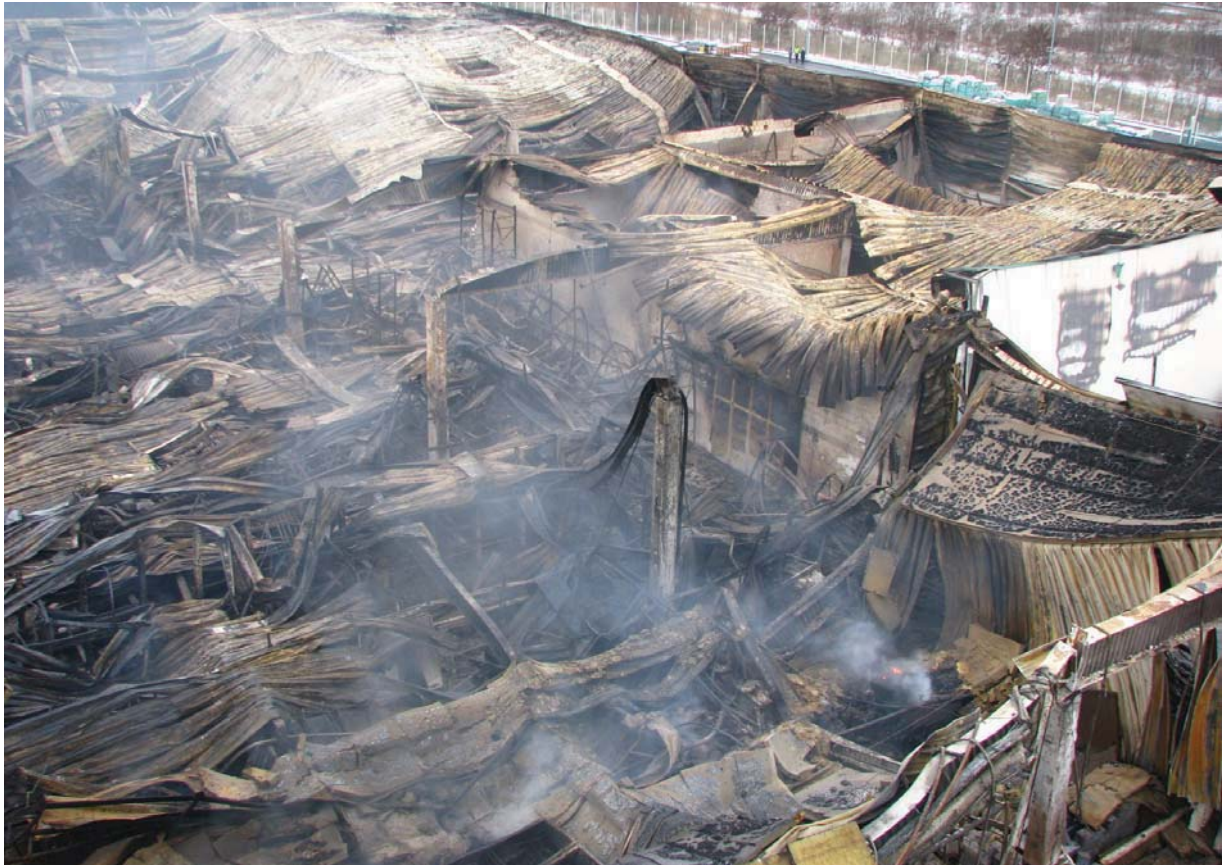
Fig. 11.1 General view of burned commercial building
