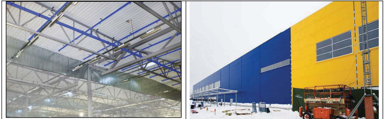
Fig. 10.2 Sprinkler protection network on the left. Building site on the right
