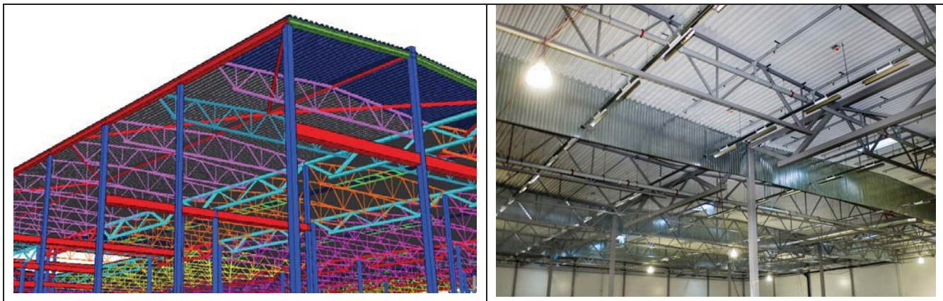
Fig. 10.1 Part of the frame system taken from Tekla Structures model and during the construction
