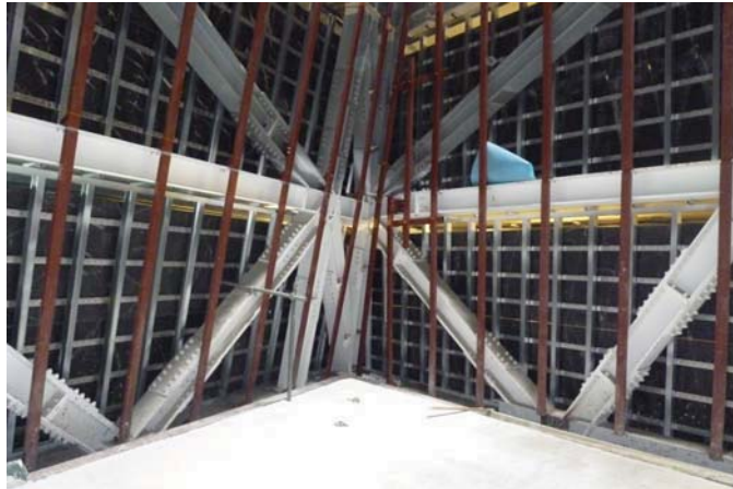
Fig. 27.14 Intumescent paint sprayed on site at first floor
