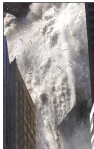
South Tower Collapsing
