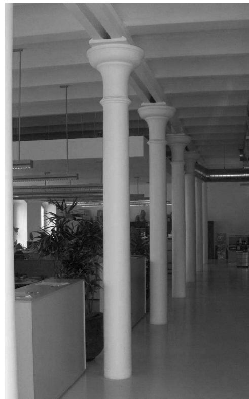
Fig. 2 Reused cast iron columns in a design office at the first floor
