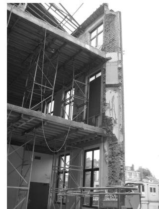
Fig. 2 View from demolished area
