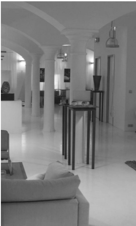
Fig. 1 Reused cast iron columns in a show room at ground floor
