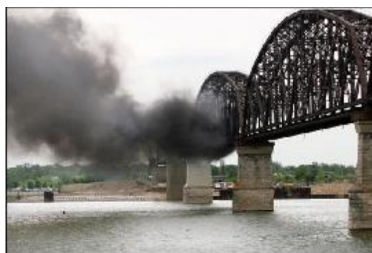
Fig. 2. Fire on the Big Four Bridge [13]
