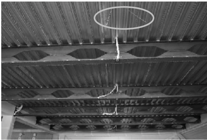
Fig. 5 Thermocouples for gas and steel temperatures
