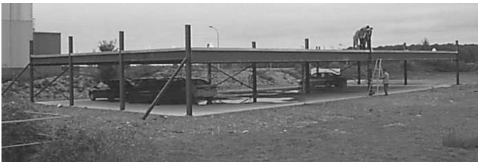
Fig. 1. Picture of the steel framed car parking under inquiry
