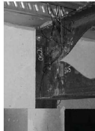
Fig. 6 Thermocouples on beam to column connection
