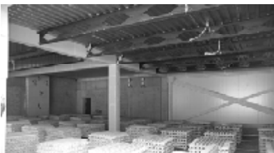
Fig. 4. Fire test set-up
